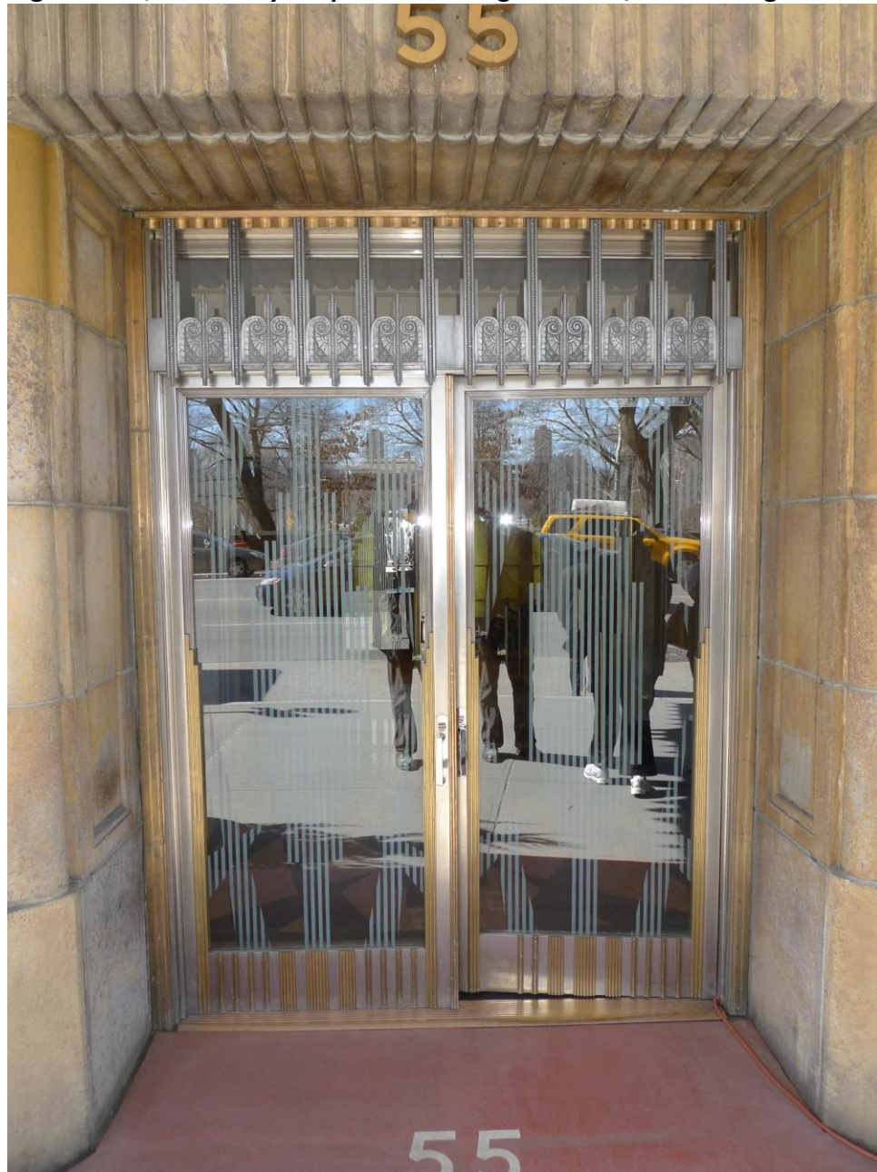
New Door astragal to left, brass "skyscraper" trim to right/ Machining trim moldings
